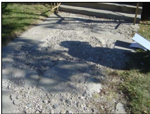
▲ Sidewalk deterioration
